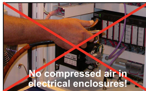
Figure 7-2: Never Use Compressed Air Inside an Electrical Enclosure
