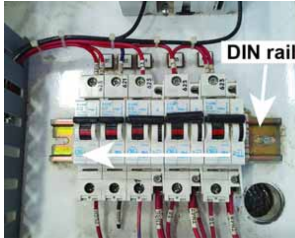
Figure 16: Shifting the Circuit Breakers
