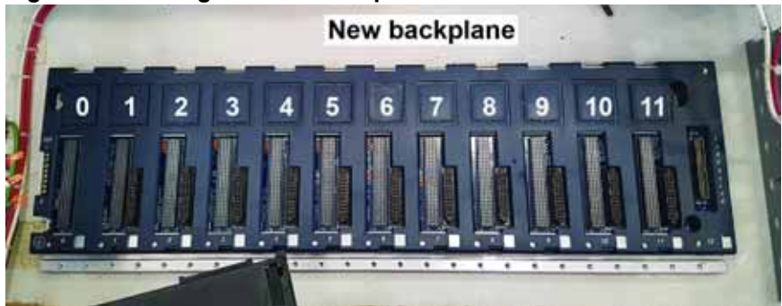
Figure 10: Placing the New Backplane
