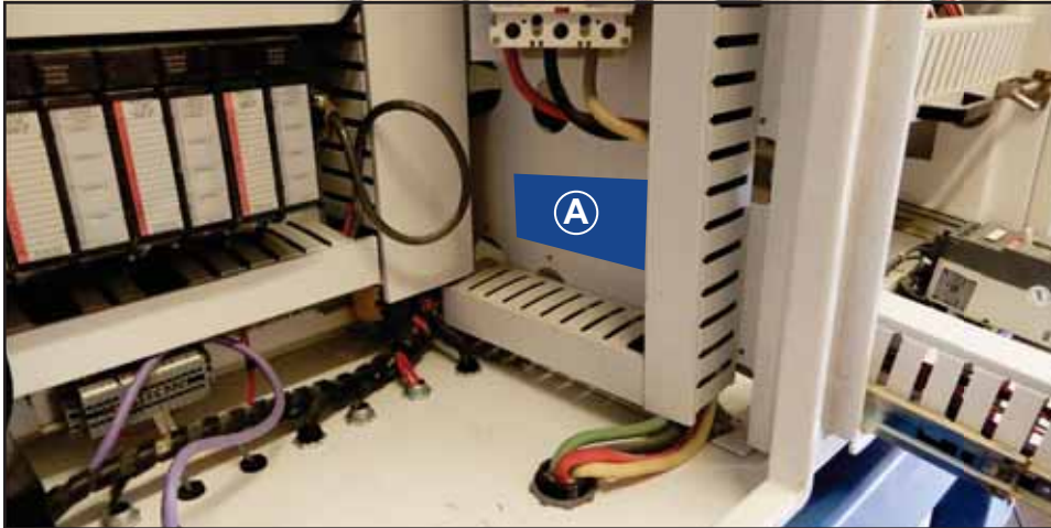
Figure 14: DIN Rail Mounting Location
