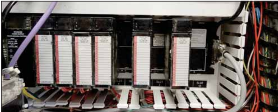
Figure 20: Carriage-End Output Modules Removed
