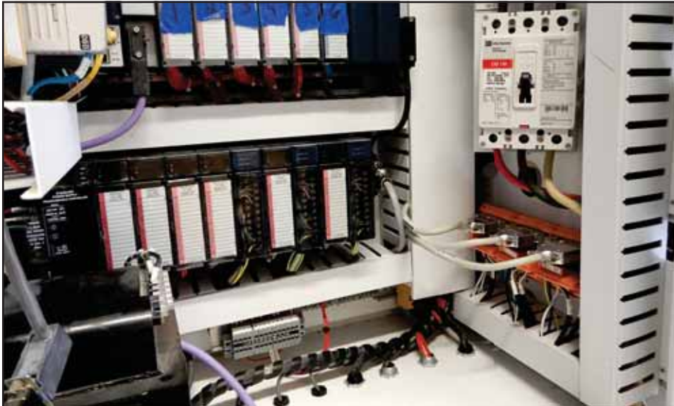
Figure 31: Stationary-End Electrical Enclosure Modules Installed
