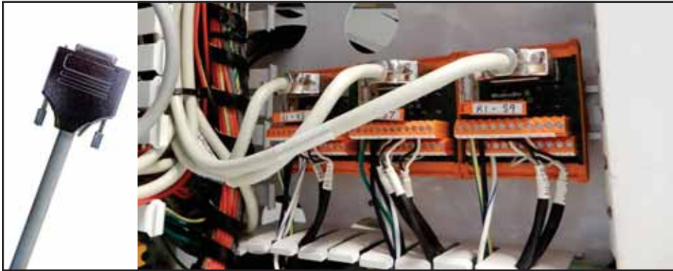
Figure 30: Connecting Interface Module End of the PAC
