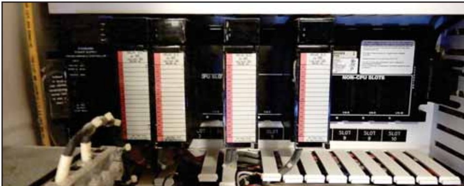
Figure 20: Carriage-End Output Modules Removed
