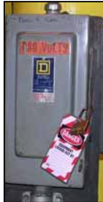
Figure SAFETY-3: Sample of a Lockout/Tagout Mechanism on a Power Source Panel
